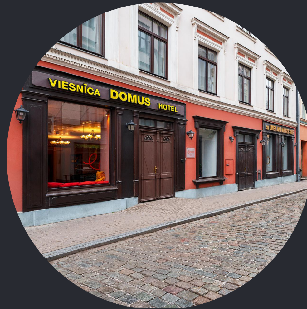
Rija Domus Hotel (under renovation)
