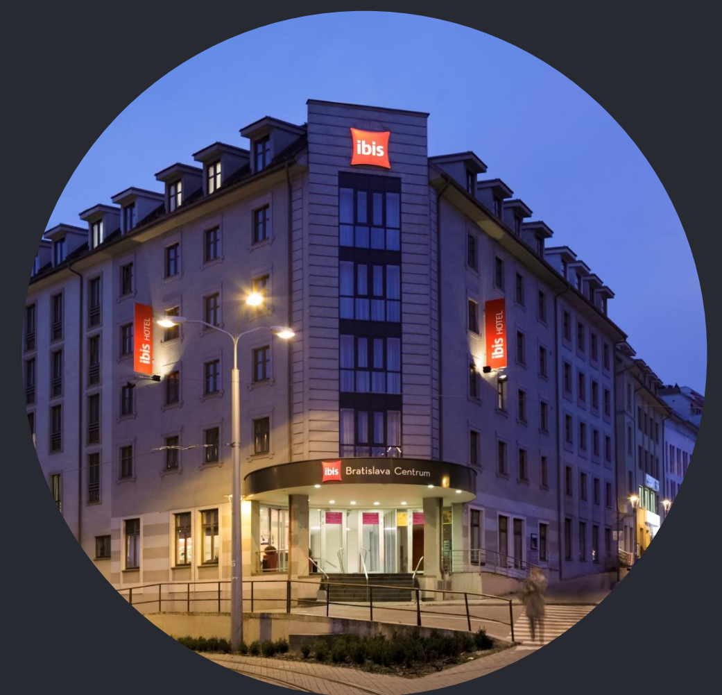
ibis Bratislava Centrum Slovakia (under renovation)
